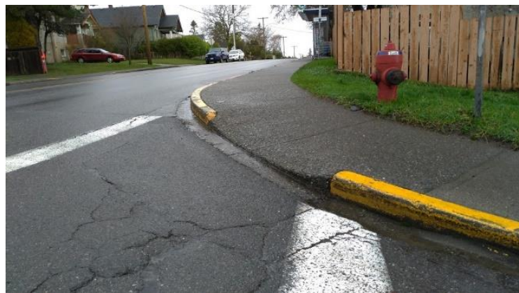
Example of deficient curb ramp in the Township.
