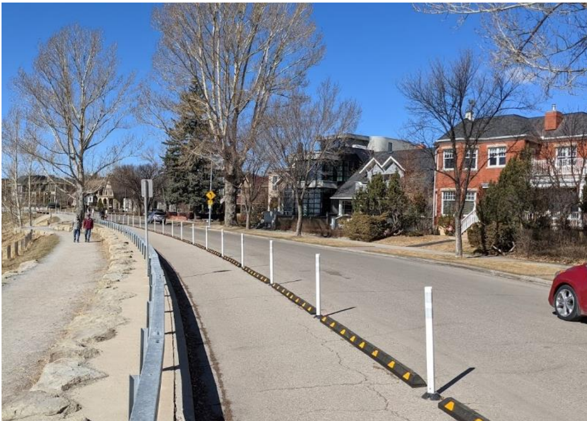
Example of a protected bike facility in Kelowna, BC with quick-build materials including flexible delineator posts and a rubber curb.
