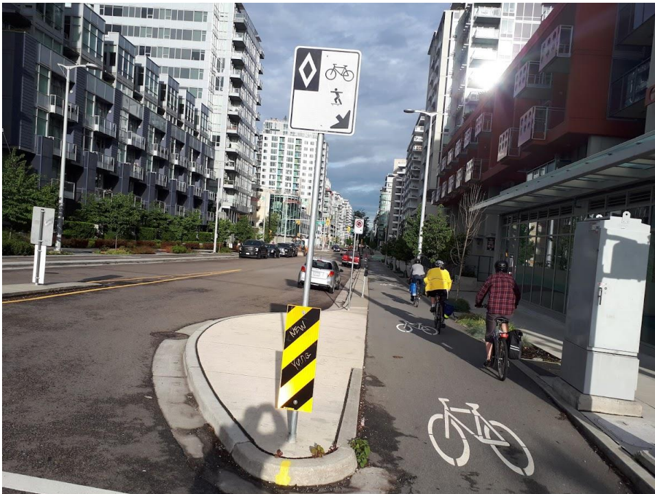
Examples of protected bike facilities in Vancouver that meet the ultimate standard. A sidewalk level protected bike lane (top) shows the bike lane separated from the road by a vertical curb and buffer.
