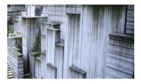
Walls are divided into two types: 1) primary walls, which are prominent perimeter retaining walls, and feature walls within the plant; and 2) secondary walls, which serve as infill between the primary walls.
