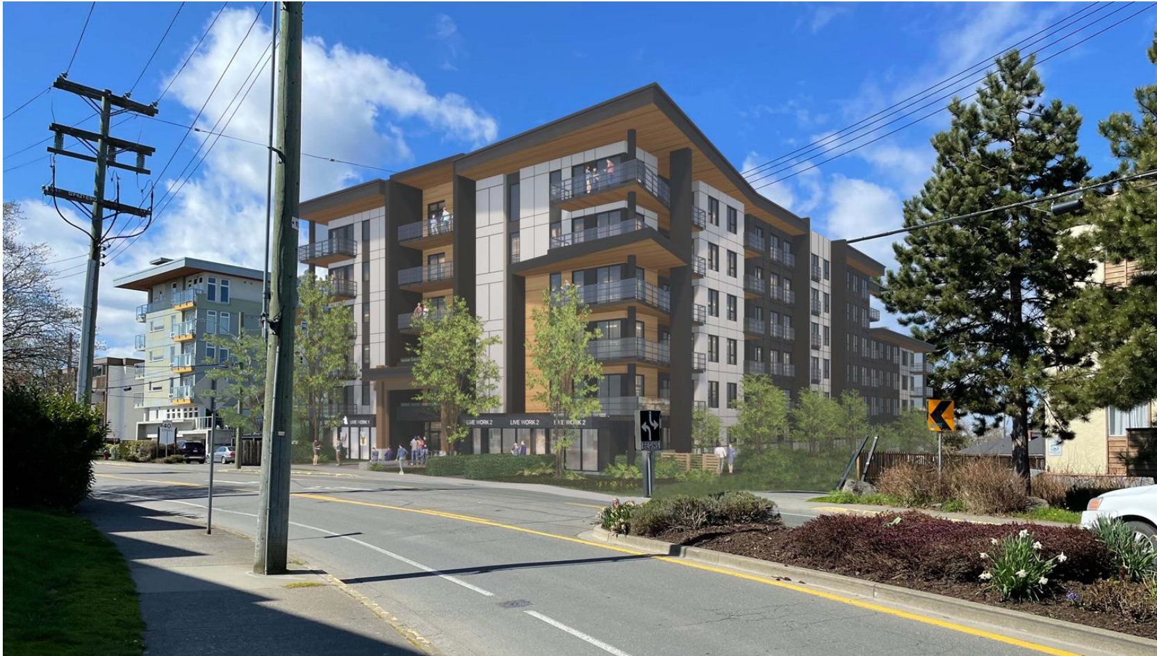
View from across the street – AFTER
