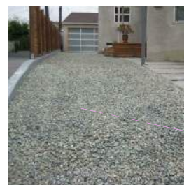
L2 COMPACTED PEA GRAVEL WALKWAYS TO REMAIN. TO BE EXTENDED TO PROPOSED PRINCIPAL BUILDING #2.
