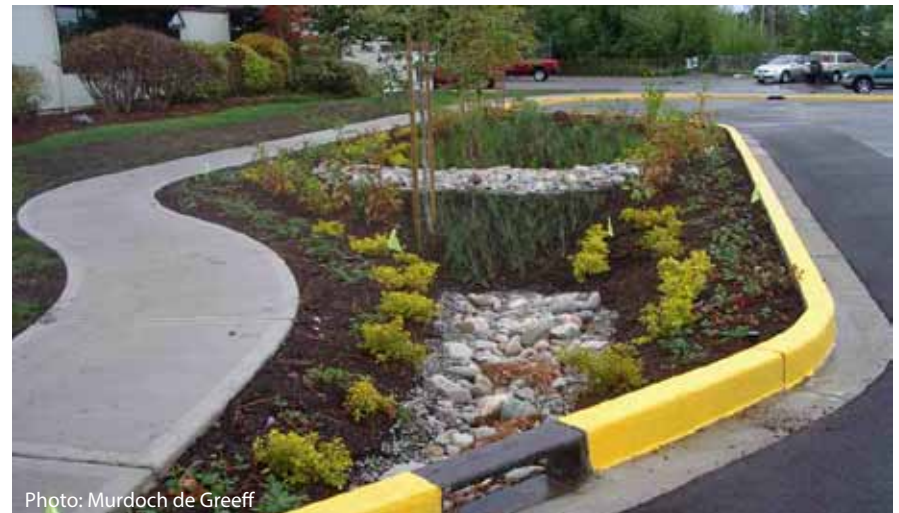
Storm Water Traffic Bulge, Trent St., Victoria BC
