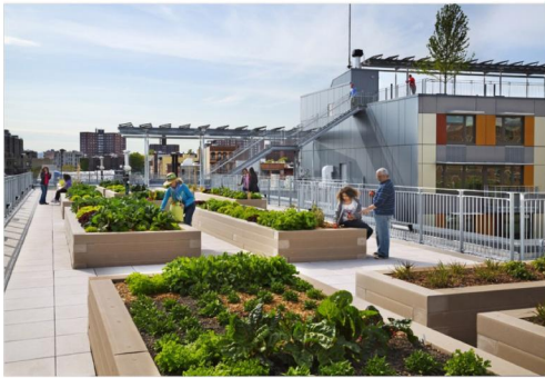
Concrete pavers on pedestal system (Typical for rooftop patios)
