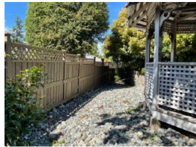
EXISTING GAZEBO TO BE REMOVED
