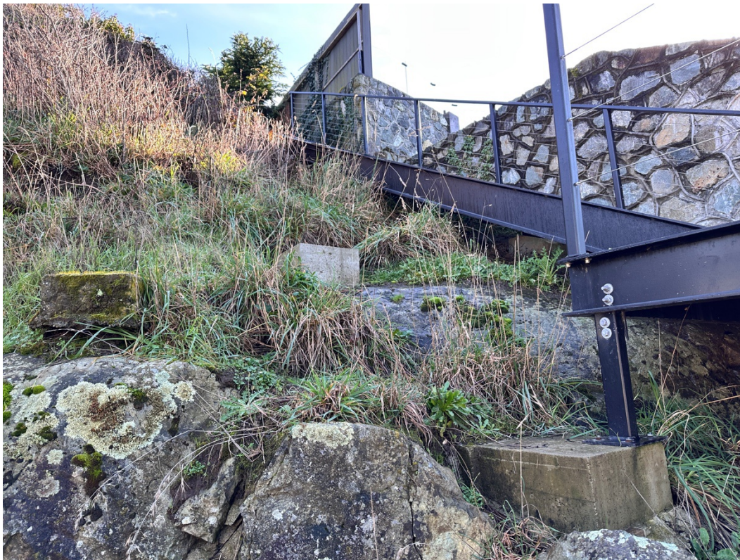
Photo 5. New landing and stairs installed between 2023 and 2025.
