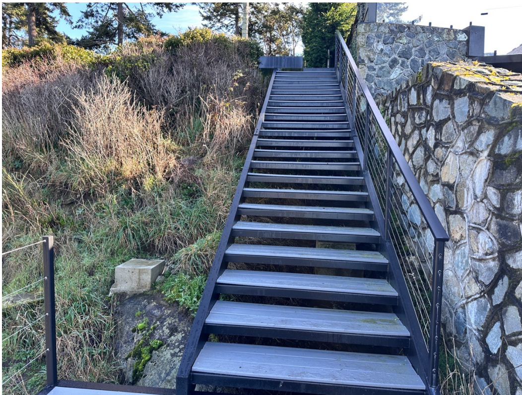
Photo 4. New landing and stairs installed between 2023 and 2025.
