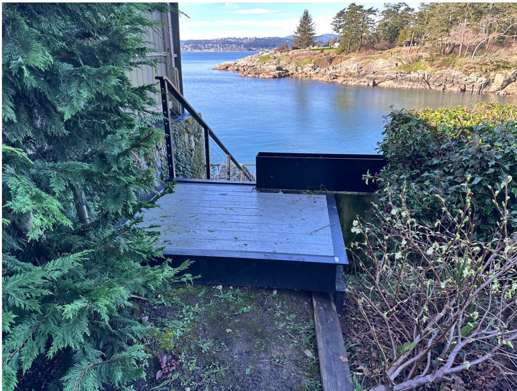
Photo 2. New landing and stairs installed between 2023 and 2025.
