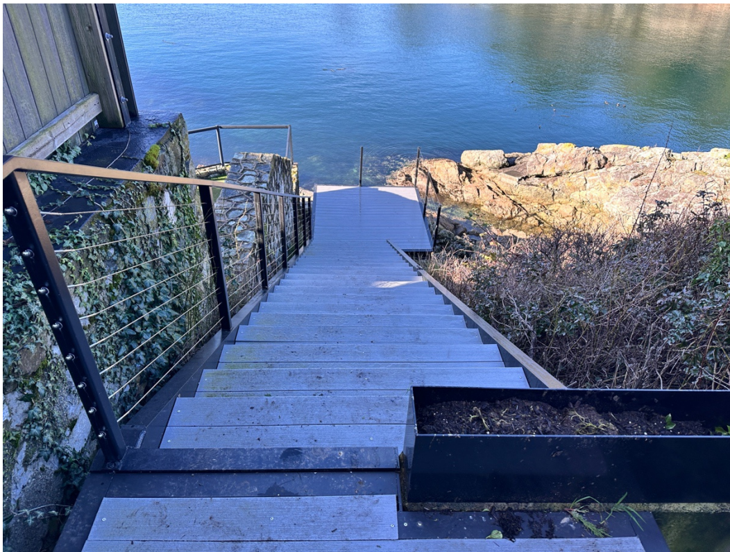
Photo 3. New landing and stairs installed between 2023 and 2025.
