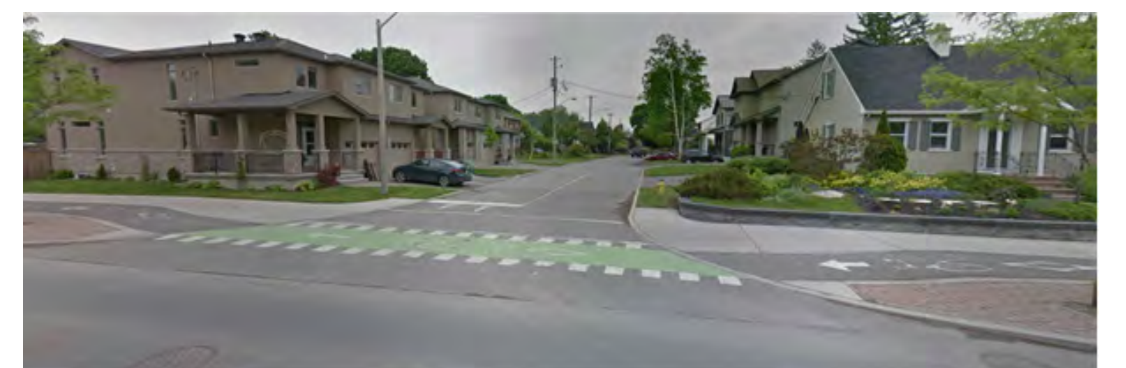
Cycle Track Treatment Churchill Ave, Ottawa
