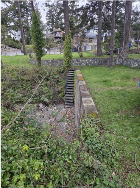
IMAGE #3: VIEW OF EXISTING RETAINING WALL. NEW RAILING FOR CODE COMPLIANCE WILL BE PLACED ON TOP.
