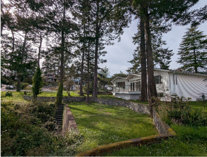
Figure 13 – View of front yard, retaining walls, and existing structure
