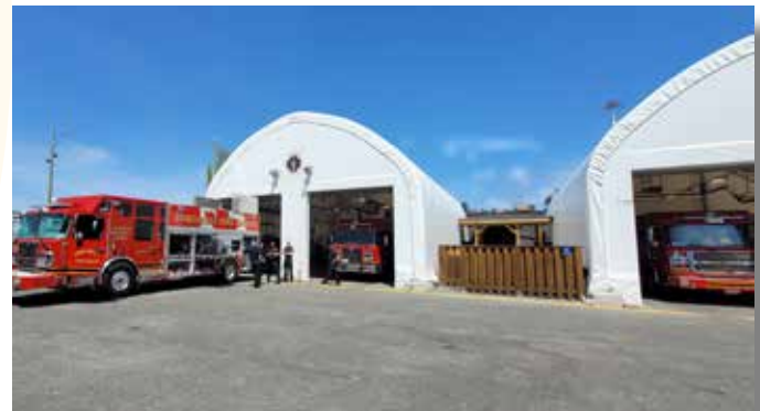
Temporary fire hall located in the Archie Browning Centre parking lot.
