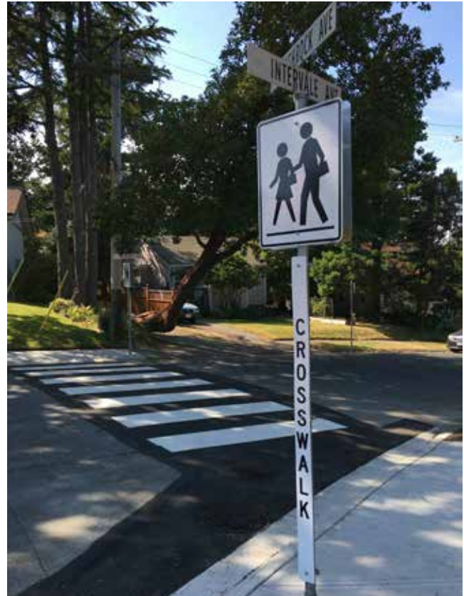
Crossing improvements at Intervale Ave and Highrock Ave, including fresh paint, new curb ramps and signage.
