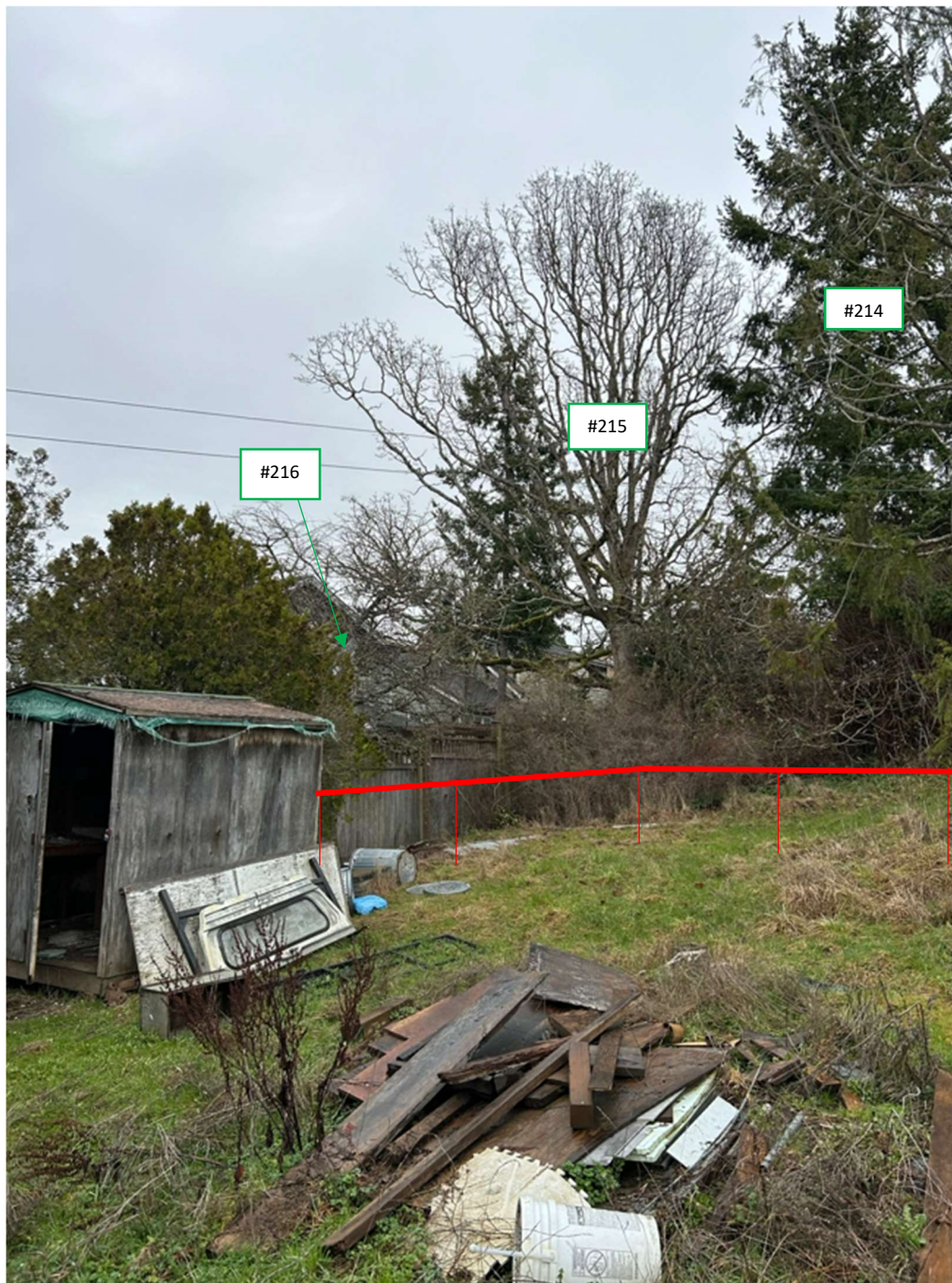
Figure 6- Northeast facing from south-central PL. Demo Phase.
