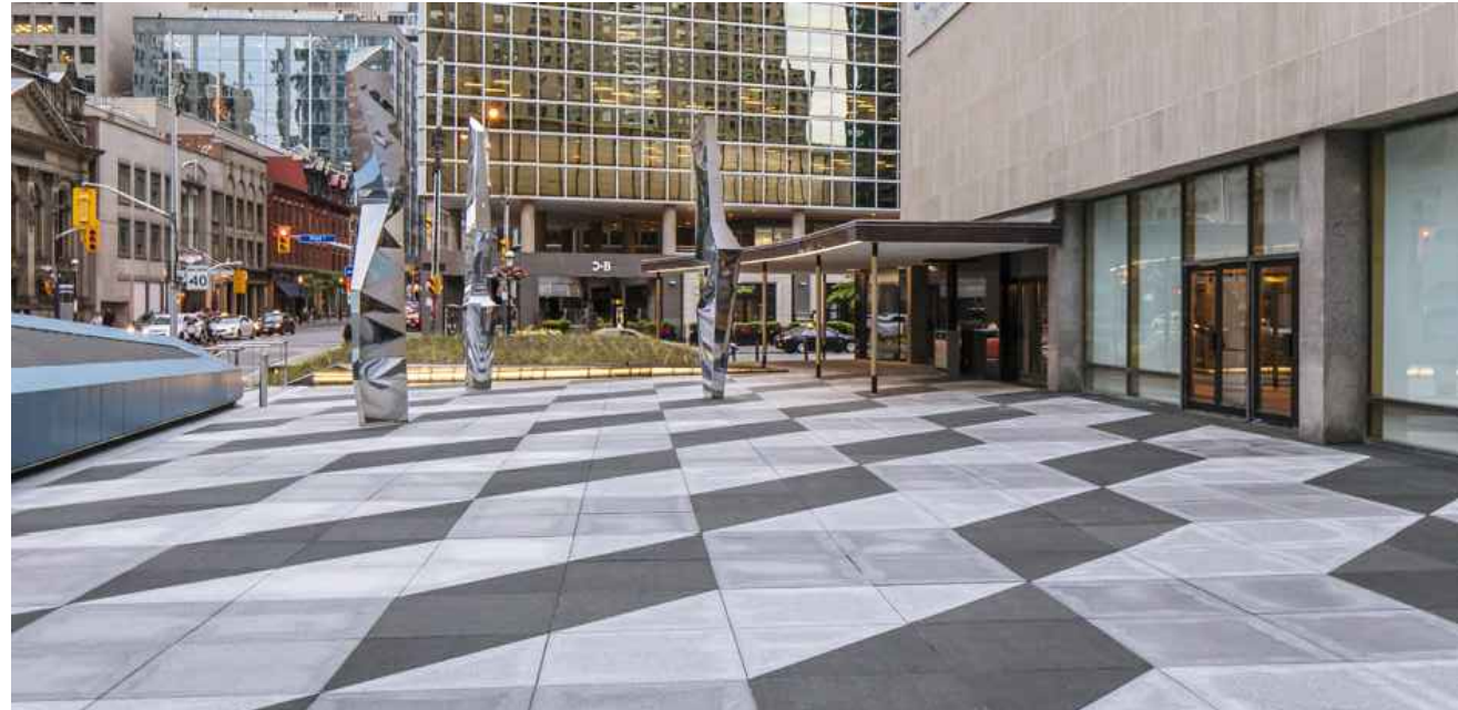
CONCRETE SLAB WITH GEOMETRIC CUT LINES
