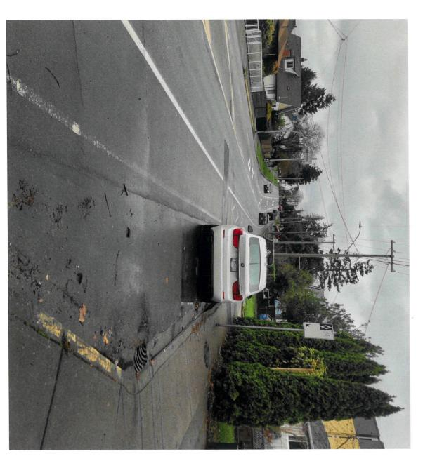
Humbolt Street Measurement: Parking/Buffer/Bike Lane 14ft/4.3m Bike Lane 5ft/1.5m Buffer 2ft/0.6m Parking 7ft
