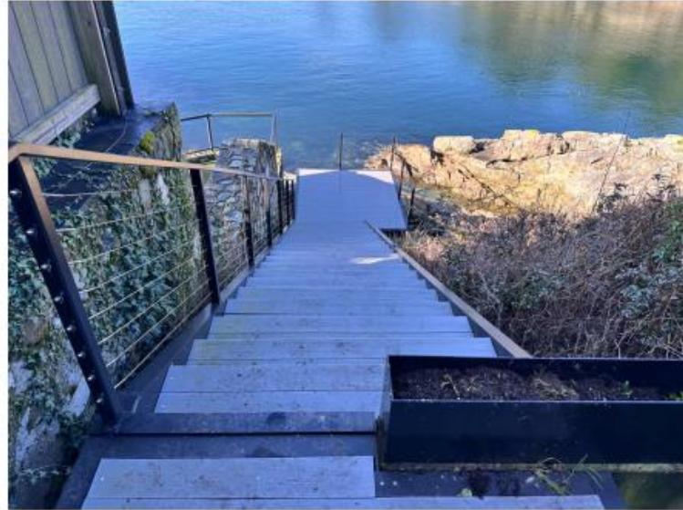
Photo 3. New landing and stairs installed between 2023 and 2025.
