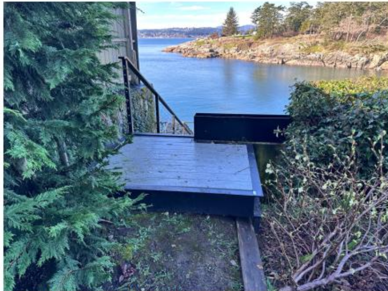
Photo 2. New landing and stairs installed between 2023 and 2025.
