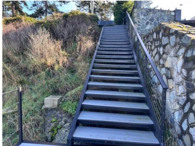
Photo 4. New landing and stairs installed between 2023 and 2025.
