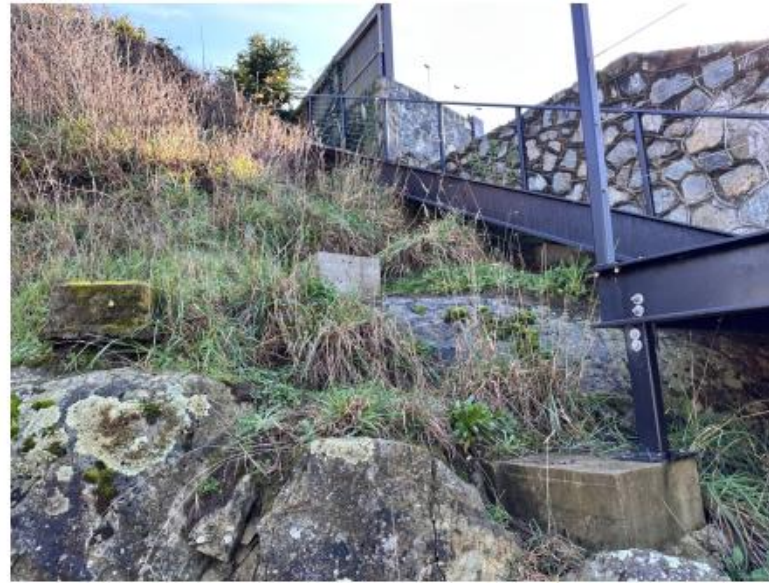
Photo 5. New landing and stairs installed between 2023 and 2025.
