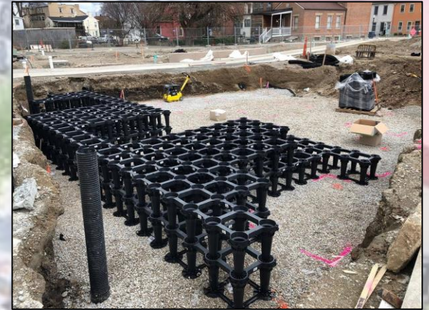
Soil Cell Installation
