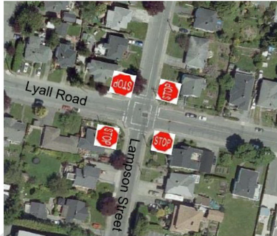
Figure 14: Existing Lampson Street / Lyall Road Intersection
